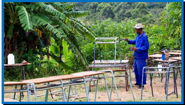
Apprentice painting a desk frame during the repairs at Franson Primary School
